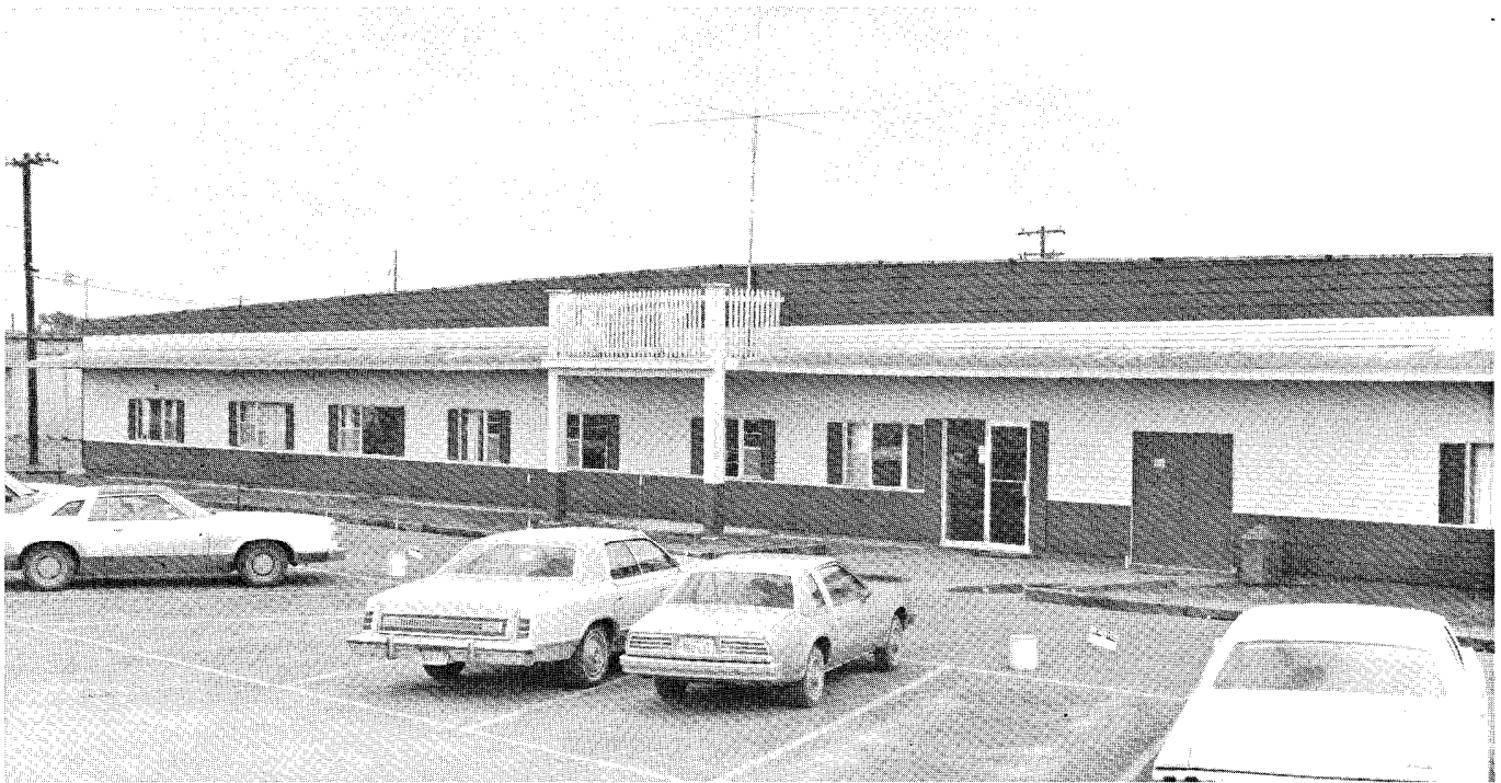
Amplifone's main office at the Brownsville complex.
