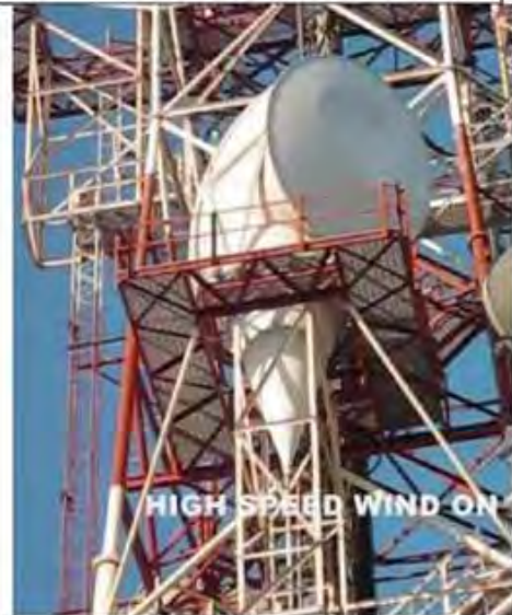
Large microwave dishes for broadband relay. Note that whip antennas are found in both residential and industrialized areas.
