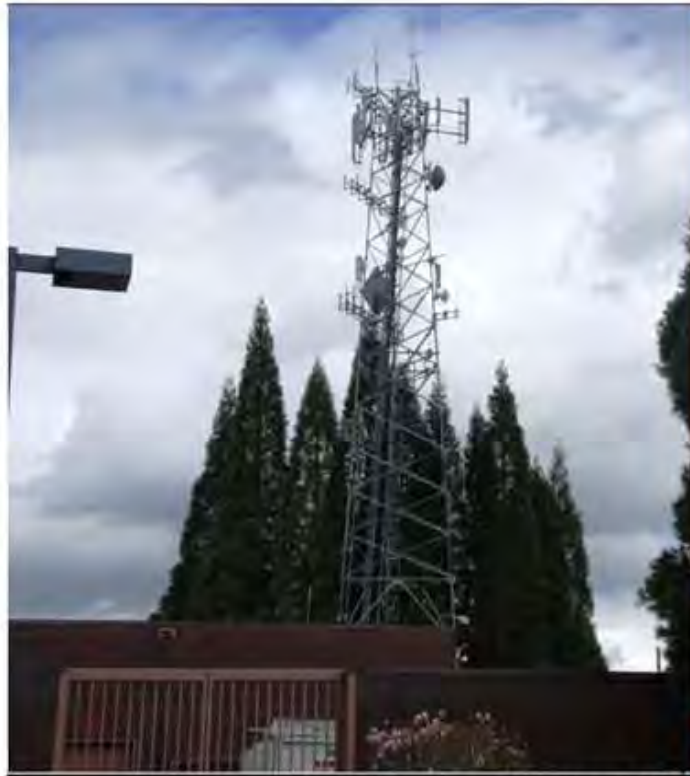
Self-supporting lattice tower with 800 MHz trunked system for most of the public safety agencies in a county and surrounding areas, including microwave links
