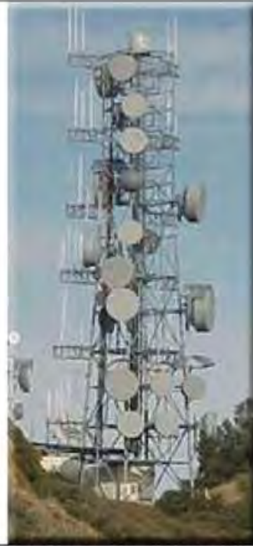
Large microwave dishes for broadband relay. Note that whip antennas are found in both residential and industrialized areas.
