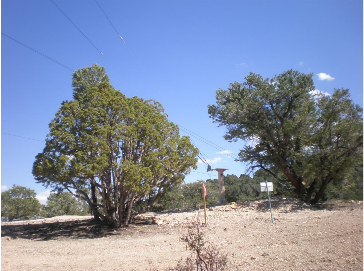
Exhibit C: Guy wire in violation of easement codes.
