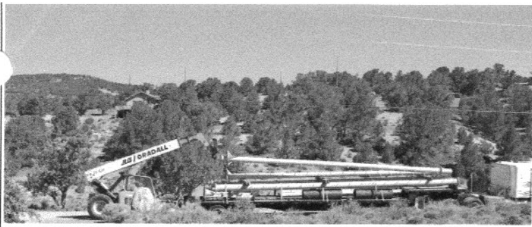
Tower is delivered on June 7. First he tried to pick up a 40' joint with the forklift blades.
