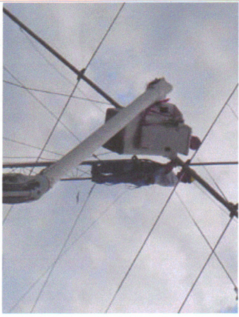
Installing the 6 element 15, July 2004
