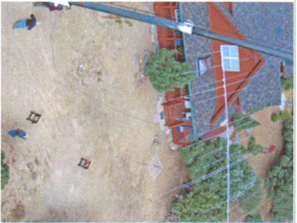
Installing the C31XR, October 2006
