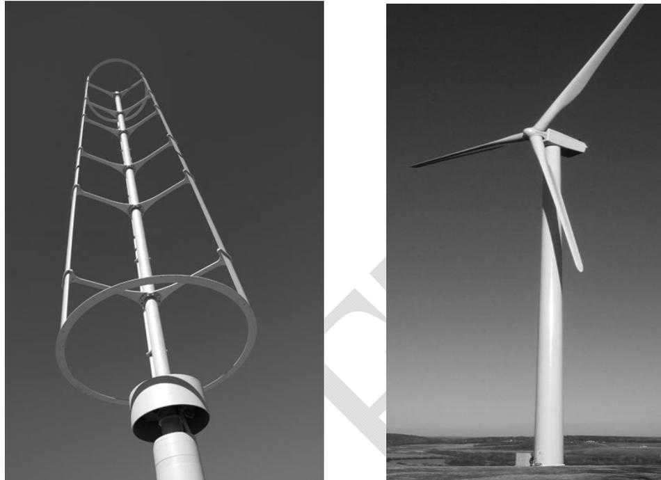
**Figure 2.2:** The Vertical Axis Wind Machine (top left) is positioned so that its main rotor shaft runs vertically to its supporting tower. The Horizontal Axis Wind Machine (top right) is positioned so that its main rotor shaft runs horizontally to its support tower. Both of the above Wind Machines are supported by a mono-pole (single pole) tower. The Wind Machine illustrated at the bottom right is supported by lattice type framework.
